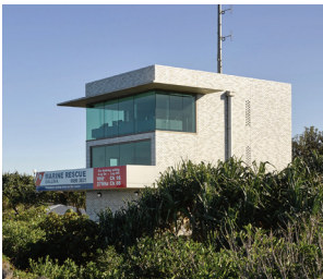
Public & Commercial Architecture Ballina Marine Rescue DFJ Architects WINNER
